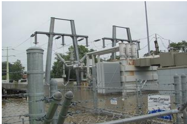
Figure 1: Flooded Substation (FirstEnergy Corp.)
